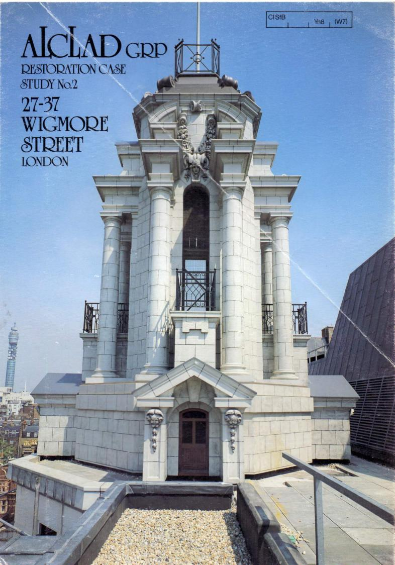
A thorough survey was carried out by Alan Butcher Associates Limited prior to the dismantling of the entire glazed terra cotta cupola and associated decorative shield and statues. Photographic records together with detailed drawings of the existing cupola were produced and some of the highly enriched features removed from site for additional reference during reproduction in Alclad GRP.
